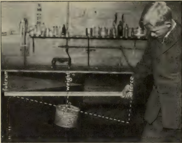
FIG. 28. A lever with the weight between the fulcrum and the force.
